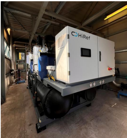
Figure 1: High temperature double effect heat pump at the Suanfarma Italia industrial facility
