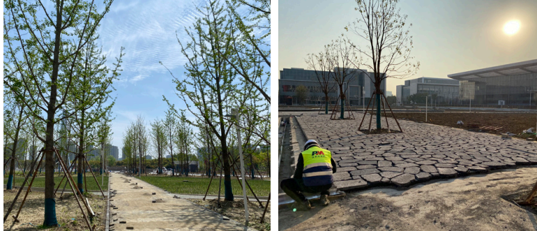
DKU Phase II construction starts in August 2019, completed in 2022 May .
