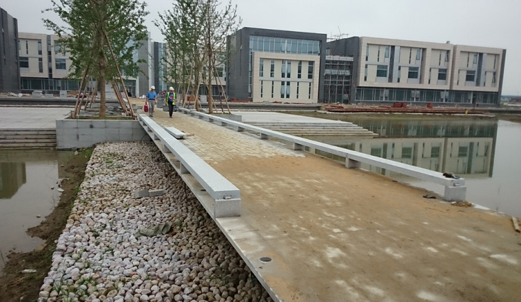
The phase I of campus construction was launched in September 2010 .
