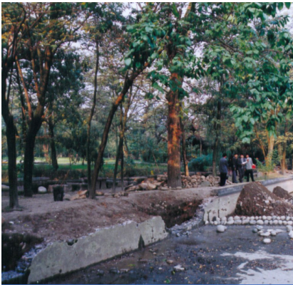
Pond: Harsh and damaged revetment curve
