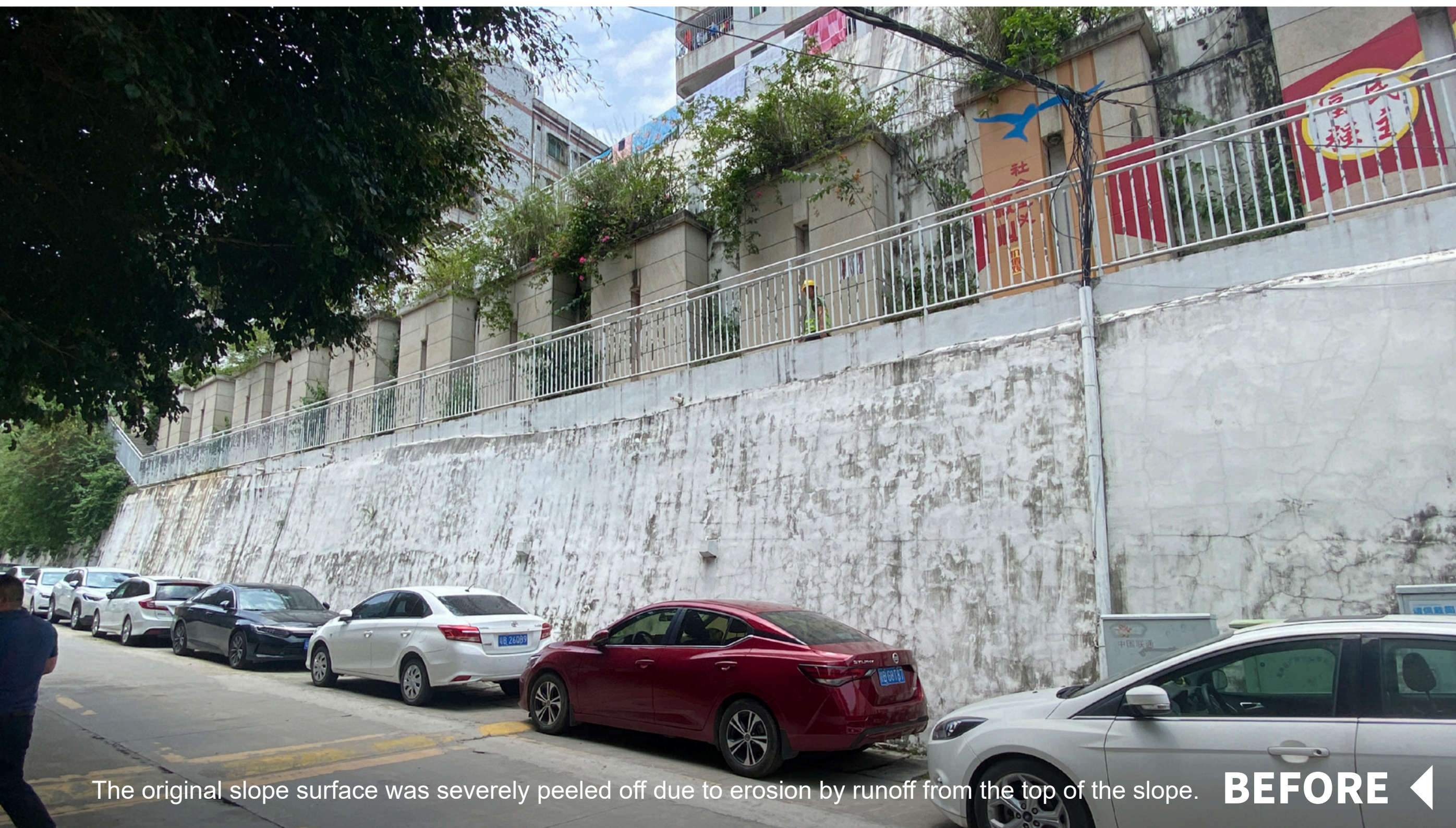
Aging external leakage drainage facilities make the retaining wall facade dirty.
