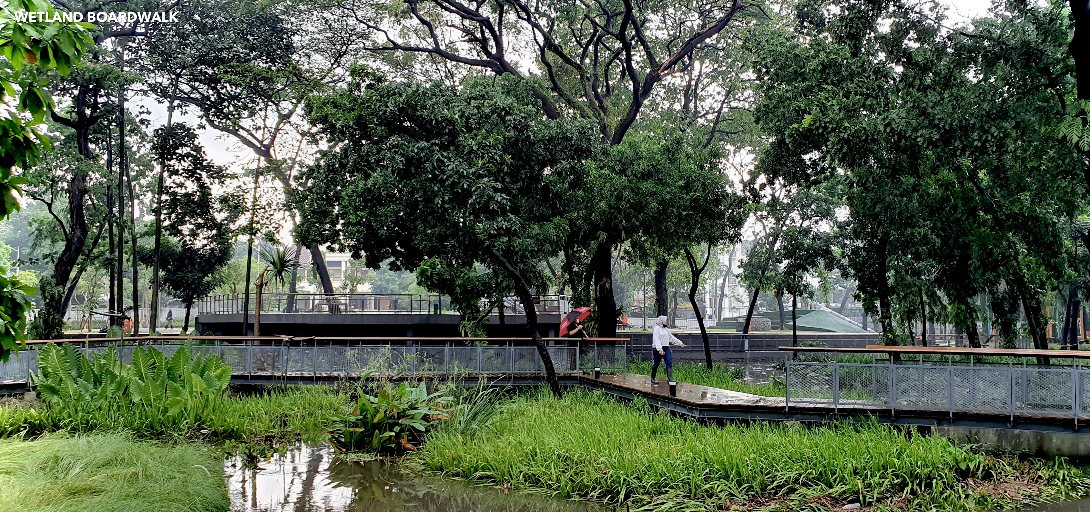
The Wetland Boardwalk is built with light construction, designed at elevation above 10 years average rainfall event, allowing pedestrian to walk through the park in wet and dry time
