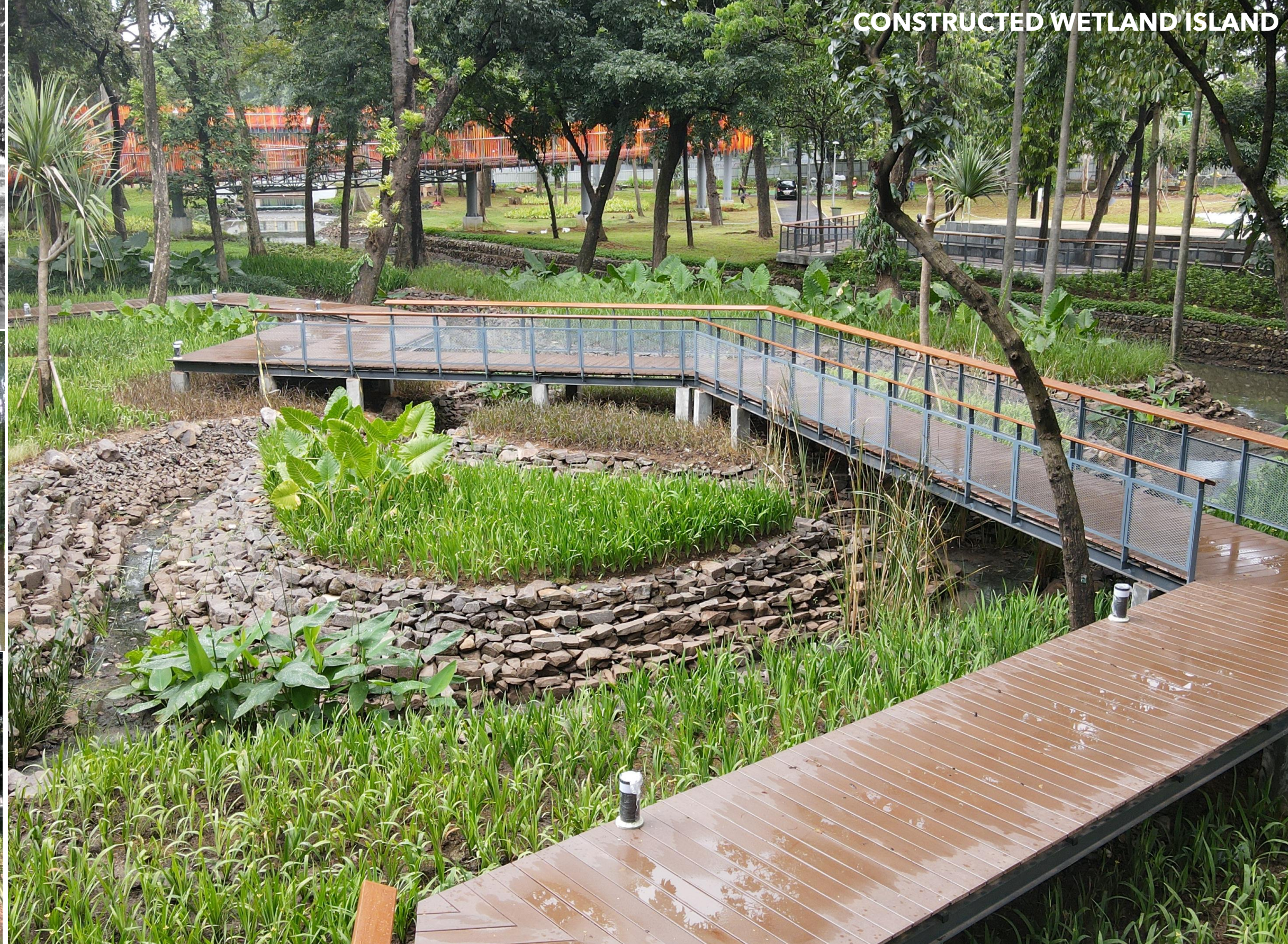
The wetland islands was built as an effective filtration and detention system for stormwater runoff to easing the park flooding while integrated with diverse array of riparian planting species to enhance aquatic ecosystems.
