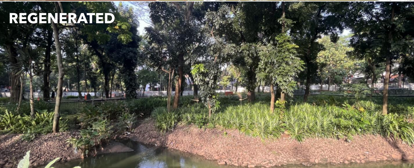
The wetland islands was built as an effective filtration and detention system for stormwater runoff to easing the park flooding while integrated with diverse array of riparian planting species to enhance aquatic ecosystems.
