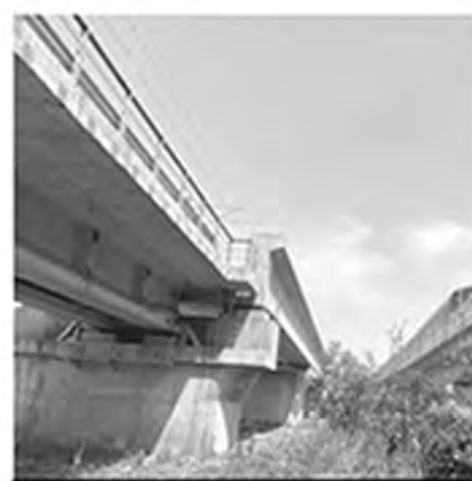
viaduct section of railway
