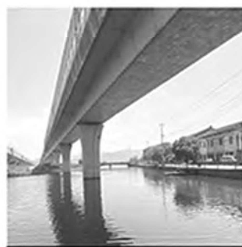
No. 1 rail line
