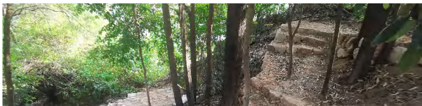
Local materials and footpaths stacked manually with stones
