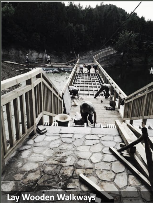
Lay A Wooden Walkway Over Ditch
