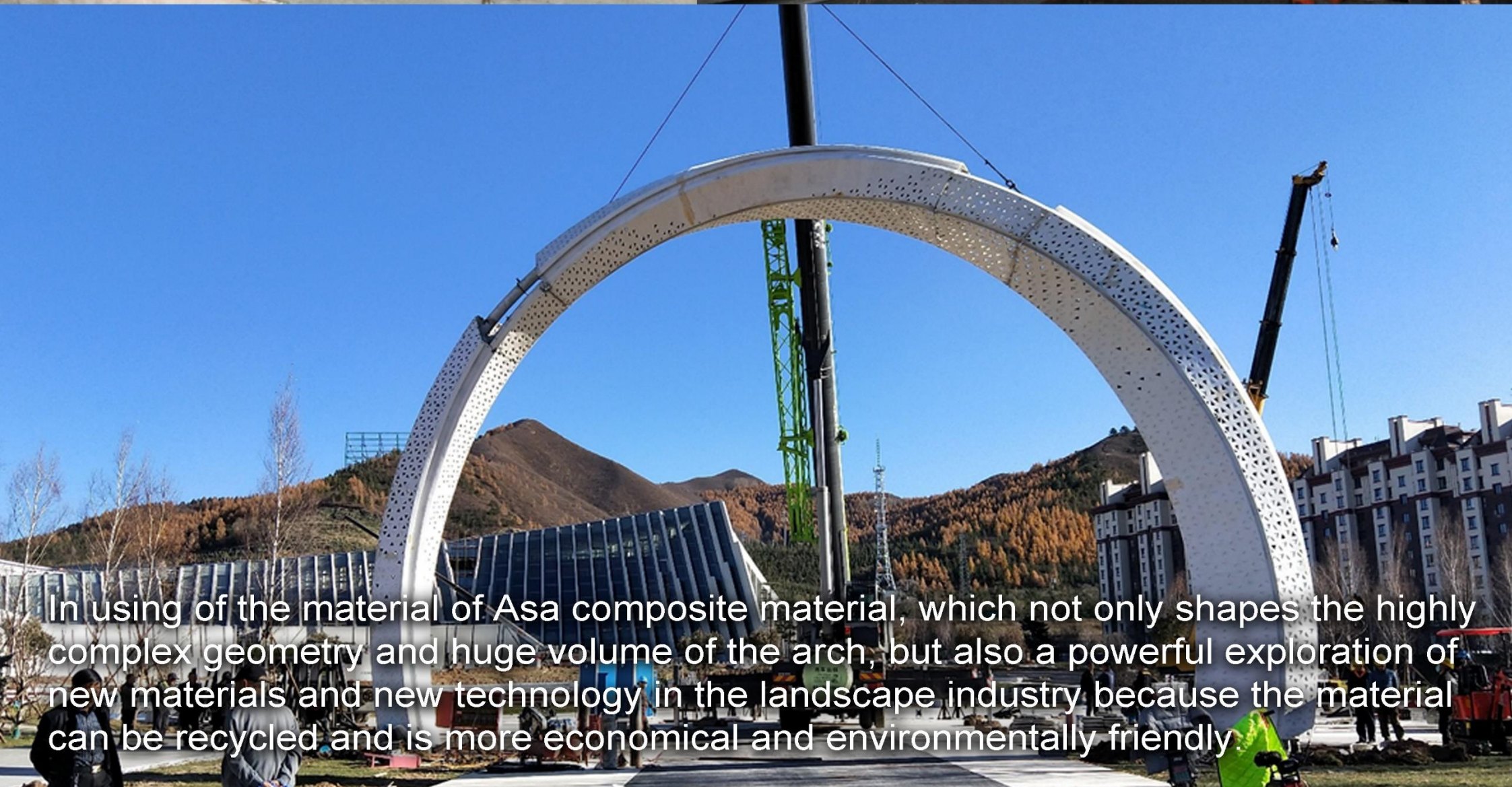
Archs are assembling with intelligent lighting system as well as structural support
