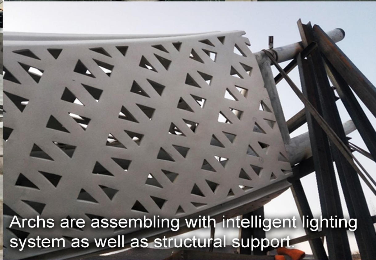
Arches are printed seperately and transported to the square site for assembling procedure.
