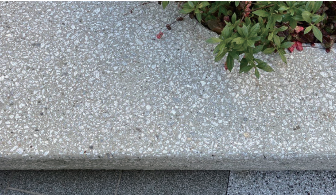
Bush-hammered concrete to conctrast with the plants
