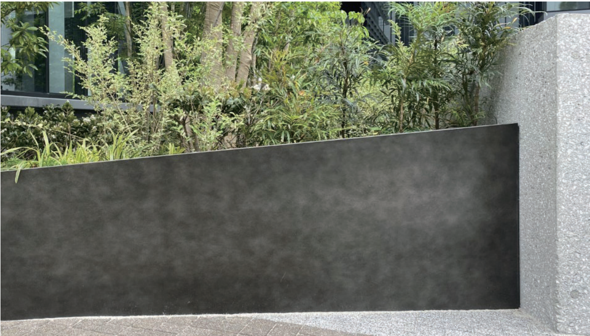
Irregular pattern finish that creates sense of depth on the steel plate
