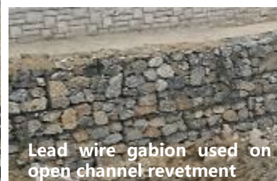
Gabion is good at rigidity and ecological compatibility, weakens the shortcomings of straight channel
