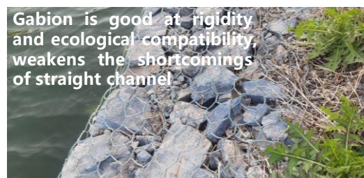
Lead wire gabion used on open channel revetment
