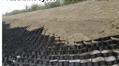
Flexible polymer honeycomb restraint system used on lake
