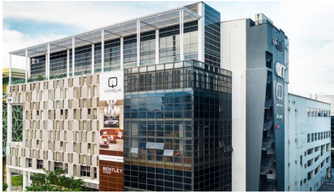
Figure 39: 16 Tai Seng St, a light industrial building, would be converted into a MTB when its master lease expires in Jun 2018
