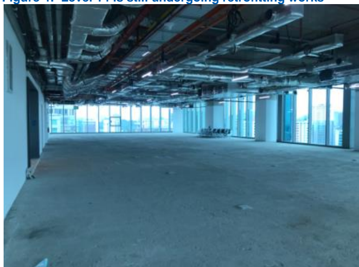
Figure 4: Level 14 is still undergoing retrofitting works
