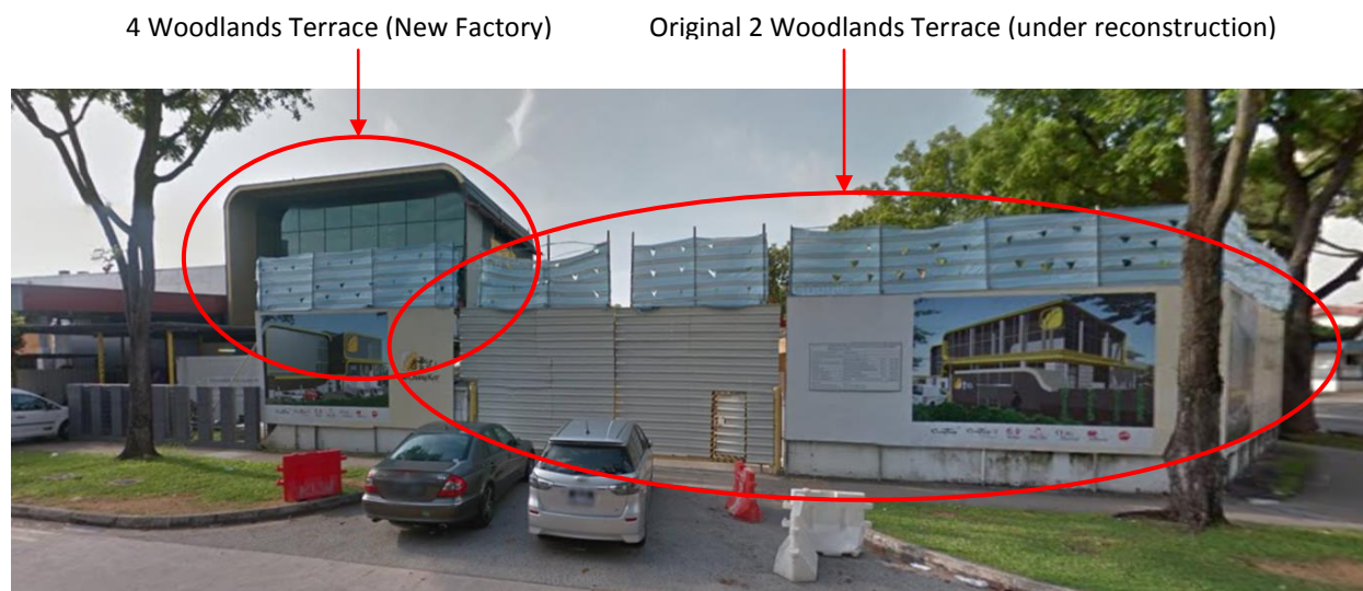
Figure 2: Factory facilities at Woodlands Terrace (as of Jul 2016)
