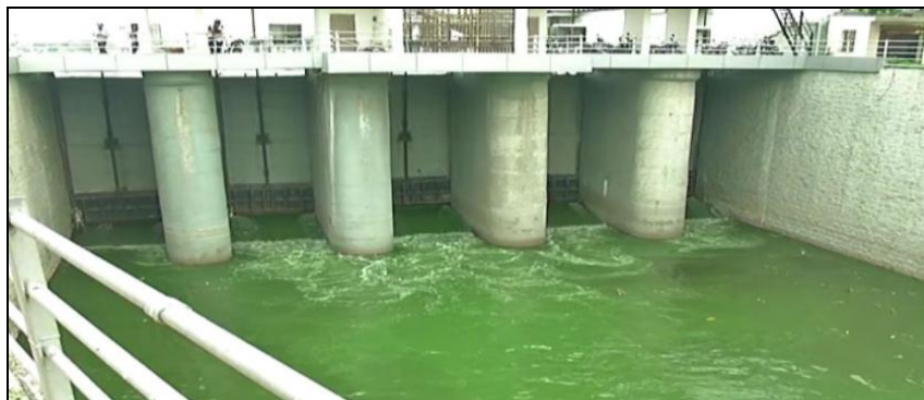
FIGURE 3.7 Fatewadi Canal of Vasana Barrage
