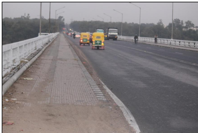
FIGURE 3.4 Chiloda Bridge on Sabarmati River (Upstream boundary)
