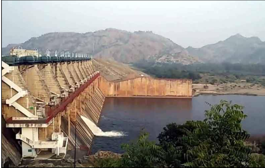
FIGURE 3.3 Dharoi Dam on Sabarmati River
