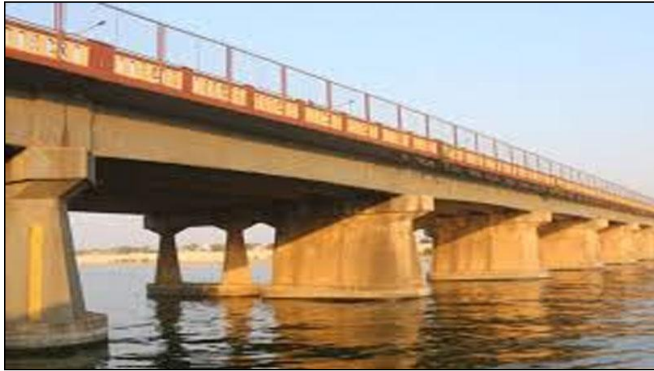
FIGURE 3.5 Subhash Bridge on Sabarmati River (Gauging site)
