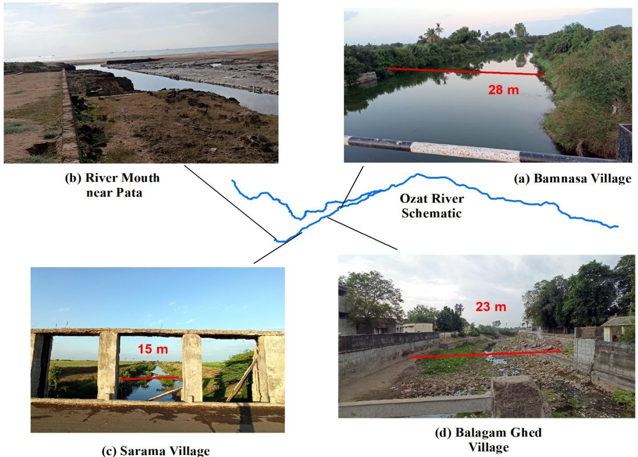
Figure 3.5 Ozat River reach (Ozat-2 Reach-1) from tikar village (bifurcation point) to river mouth near pata village
