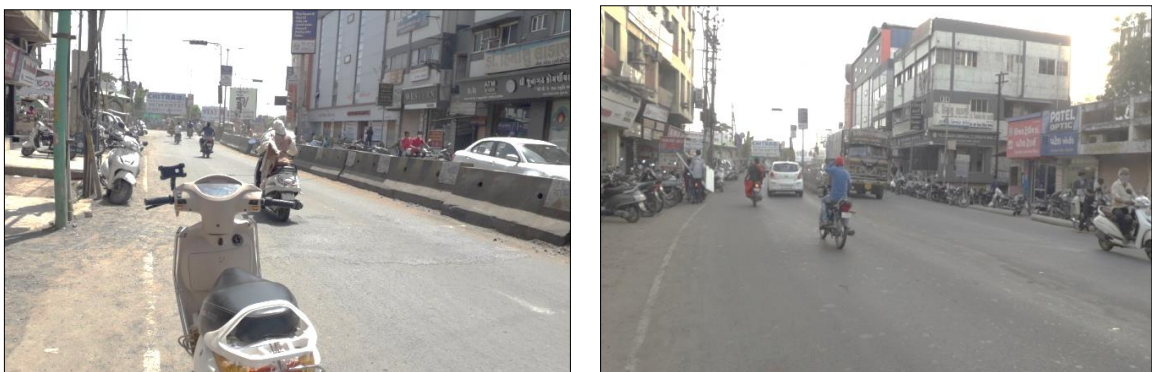
Figure 5.12 Photographs of Urban Road
