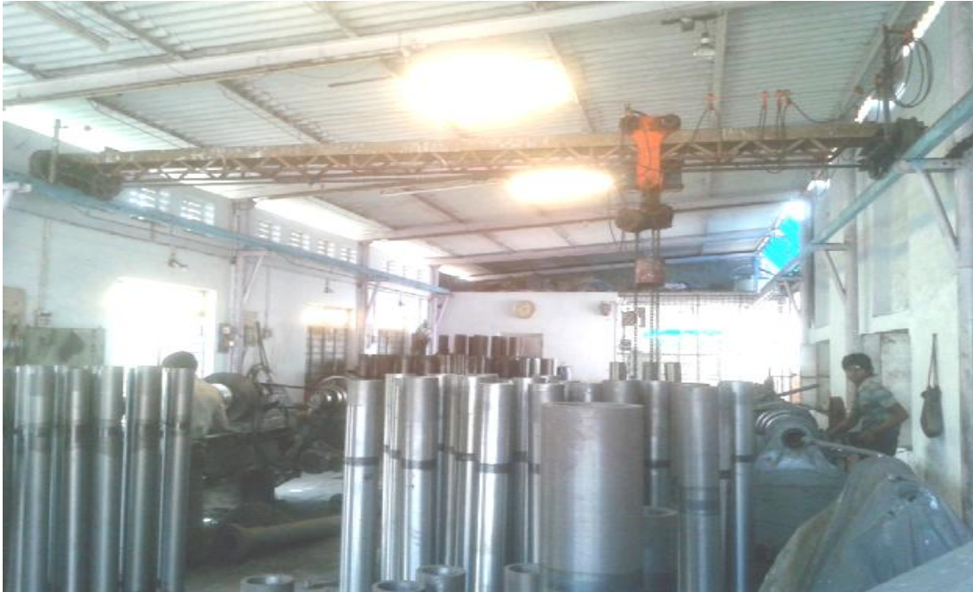
Figure 6.15. Storage of final casting pillar of drilling machine with an overhead crane in MF
