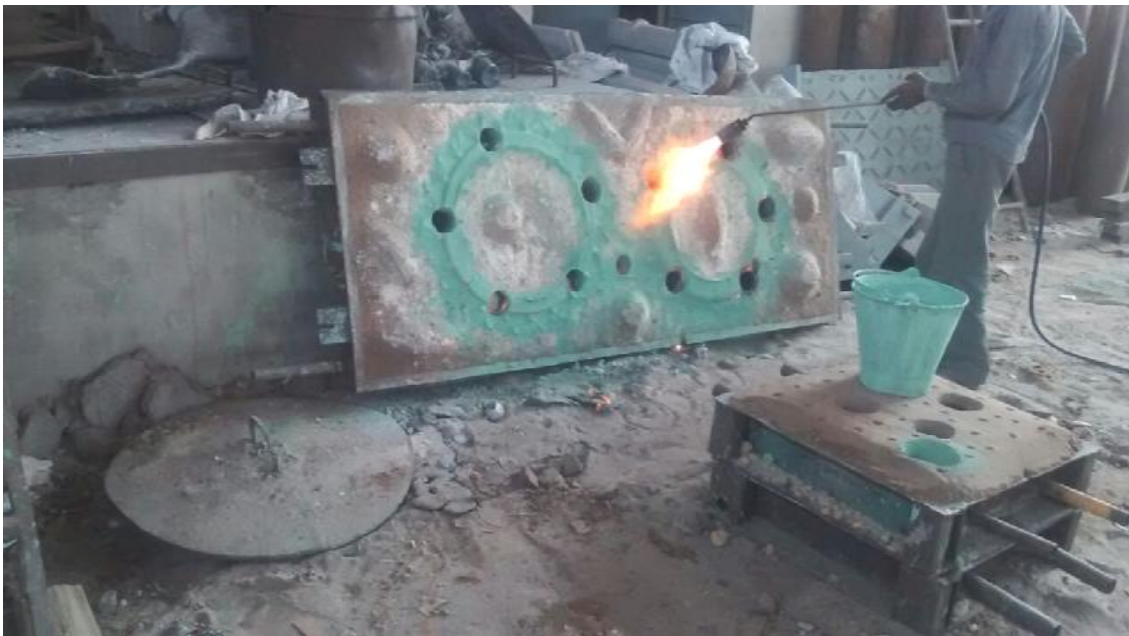
Figure 4.9. Applying Color coating on the moulds in GTC
