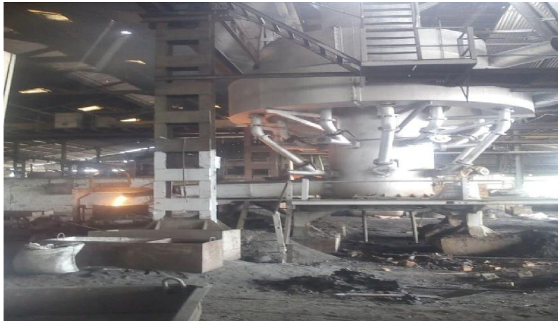
Figure 5.6 Cupola furnaces used in SF
