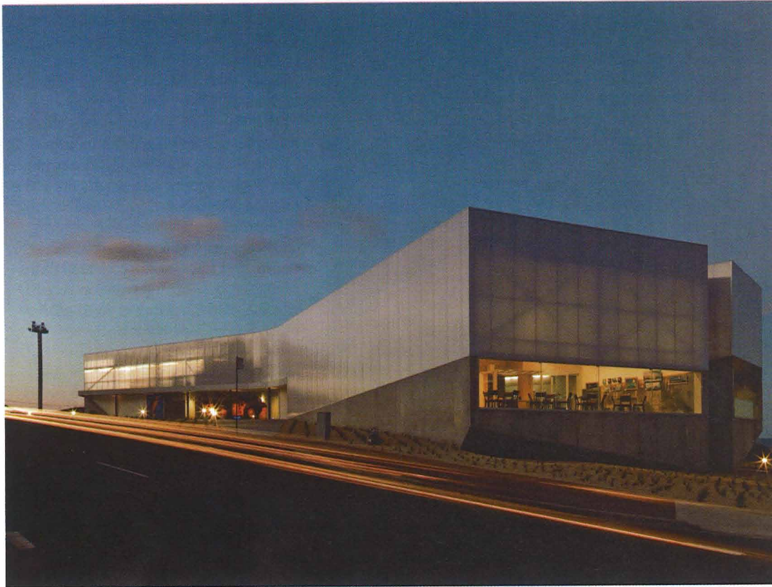
Work in progress: Architectural firm Terroir's premises in Burnie, Tasmania
