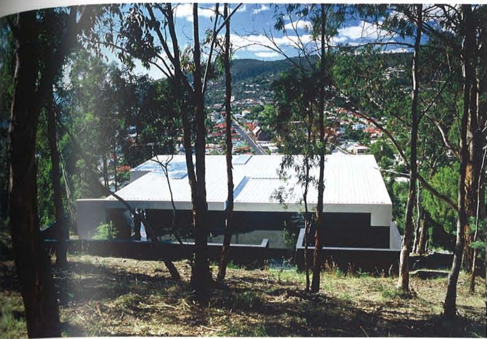
Liverpool Crescent House, Hobart, Tasmania, Australia, 2004–5. The house is a blunt cube on the exterior, with a contrastingly intimate interior. This play on contradiction is repeated in the spatial concept. Interiors are given the qualities of an exterior, for example by using zinc-coated sheet steel as ceiling linings and applying exterior render finish to interior walls. Floor-to-ceiling glazing also creates a vertiginous relation to the exterior.
